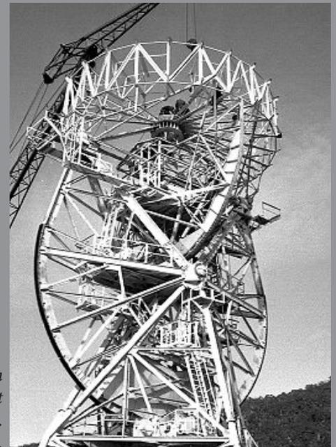
*The assembly of the parabolic dish support structure at Honeysuckle Creek.*
